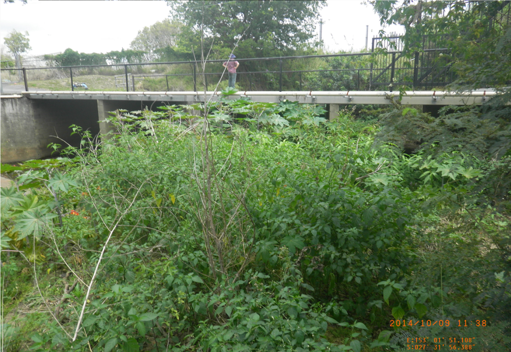
Upstream of Evesham Street Crossing
