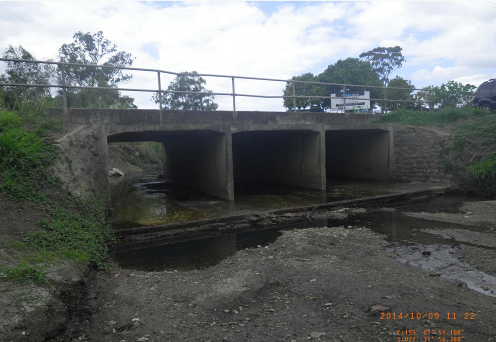
Downstream of Chale Street Culverts
