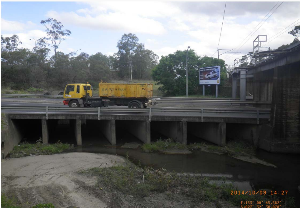
Downstream of Muriel Avenue Culverts
