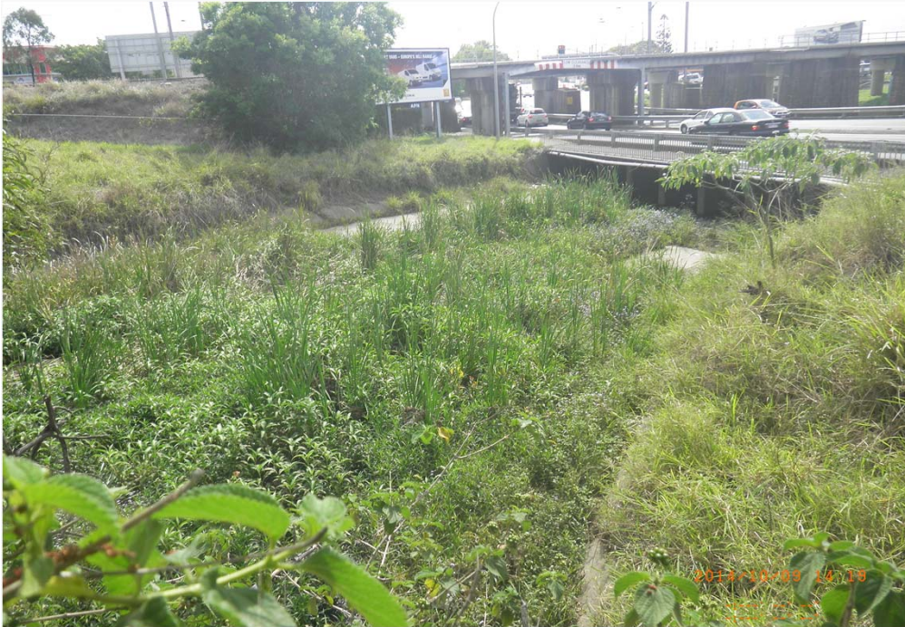
Upstream of Muriel Avenue Culverts
