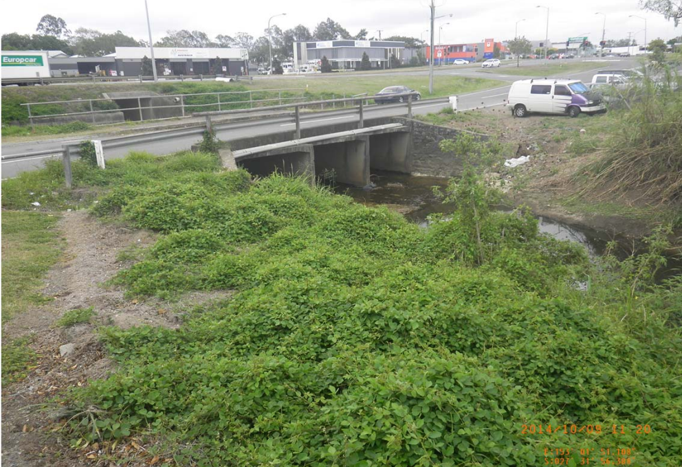
Upstream of Chale Street Culverts
