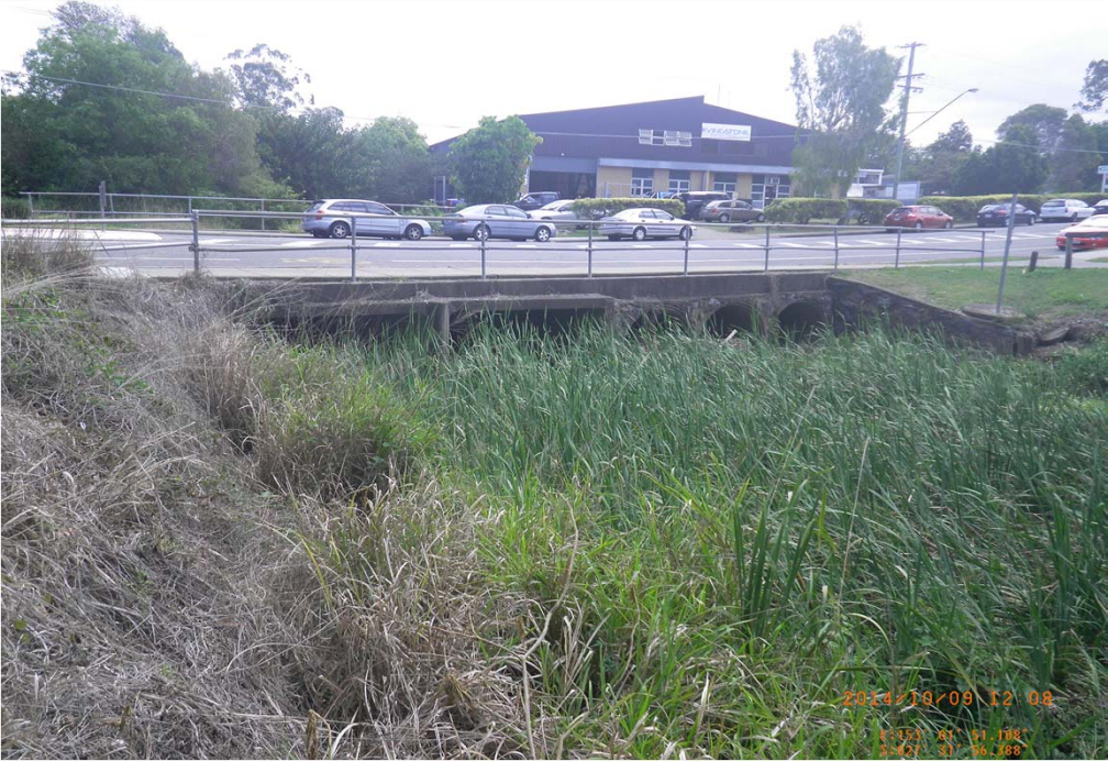
Upstream of McCarthy Road Culverts
