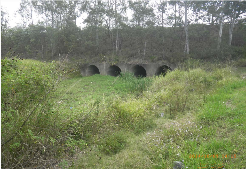
Upstream of Ipswich Road Culverts
