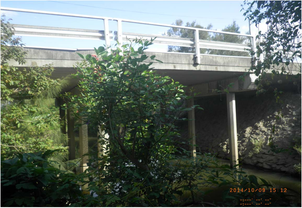
Downstream of Curzon Street Bridge
