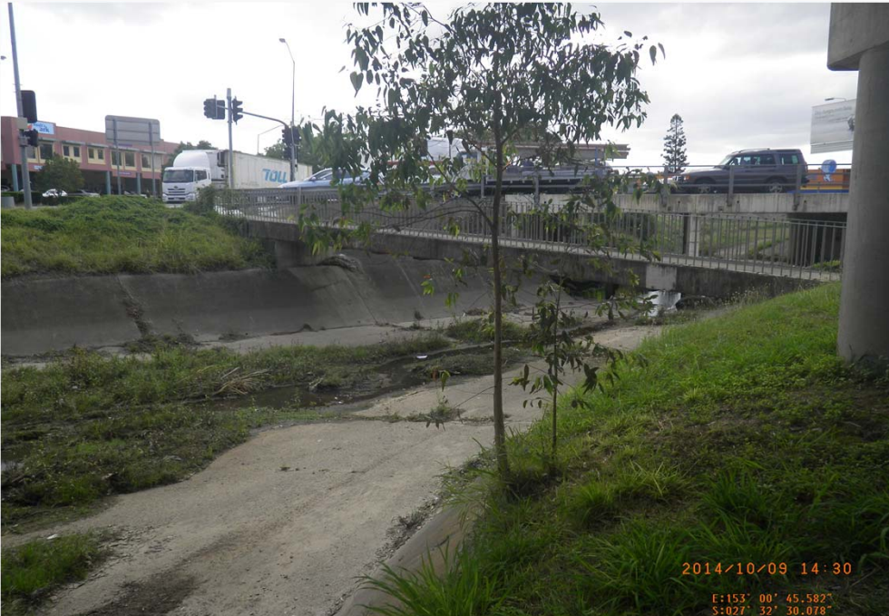
Upstream of Footbridge beside Fairfield Road
