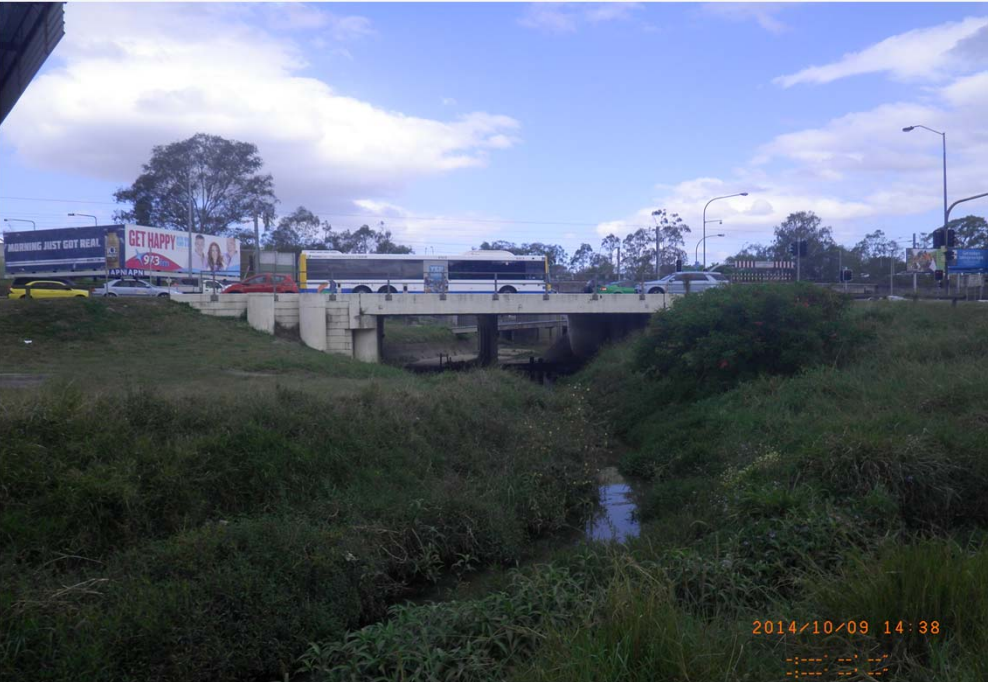
Downstream of Fairfield Road Bridge
