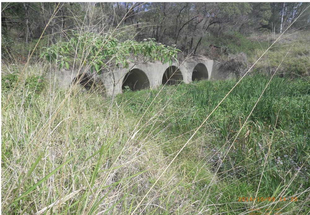
Downstream of Ipswich Road Culverts
