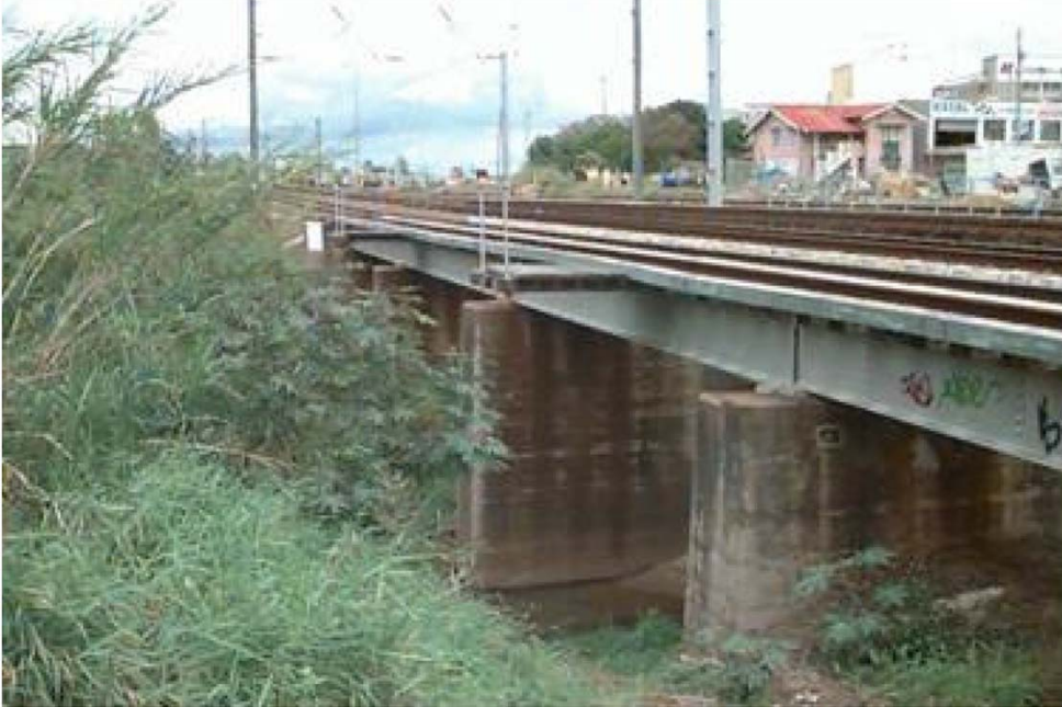
Upstream of Railway Bridges (from previous Report)
