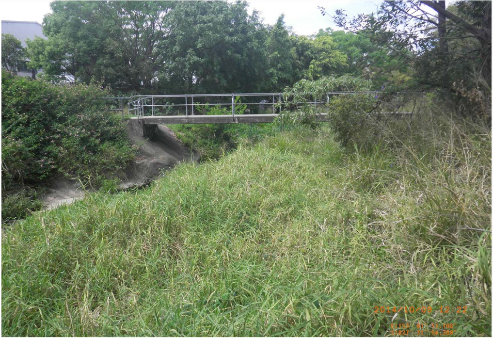
Downstream of Assembly Street Footbridge
