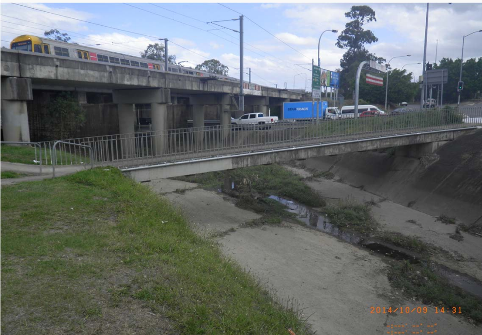
Downstream of Footbridge beside Fairfield Road
