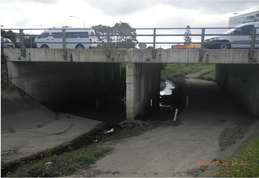
Upstream of Fairfield Road Bridge
