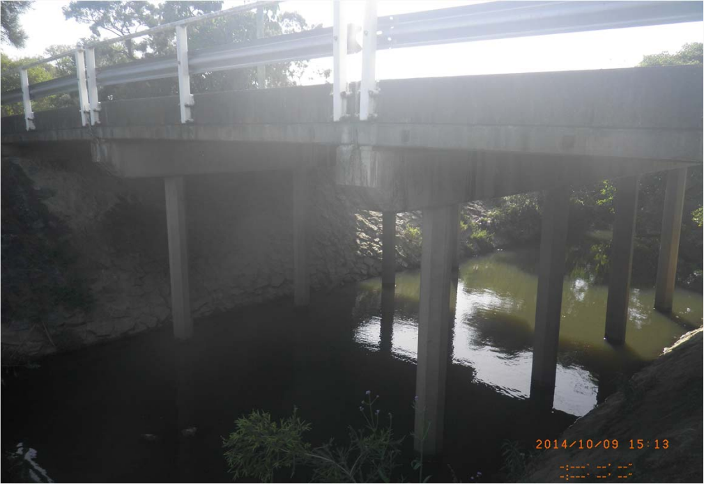
Upstream of Curzon Street Bridge
