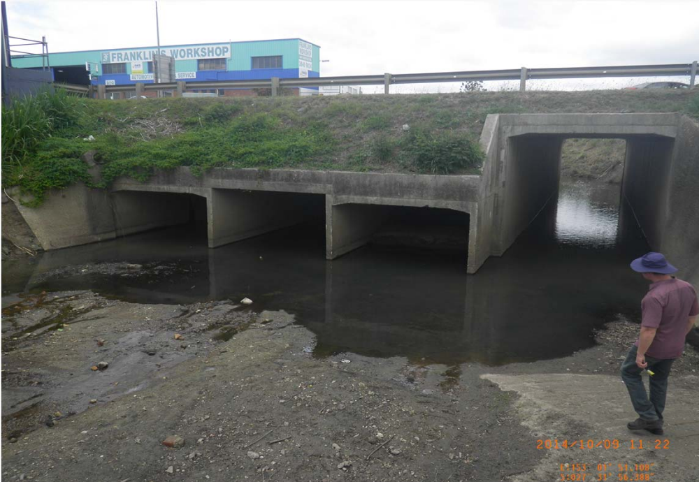
Upstream of Fairfield Road Culverts
