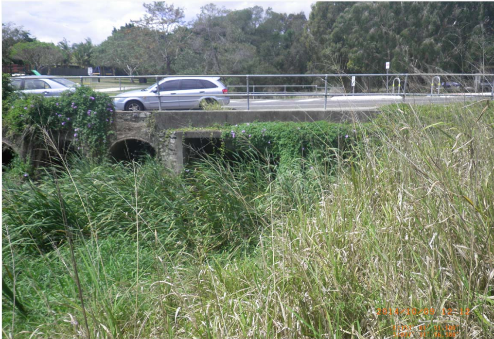
Downstream of McCarthy Road Culverts
