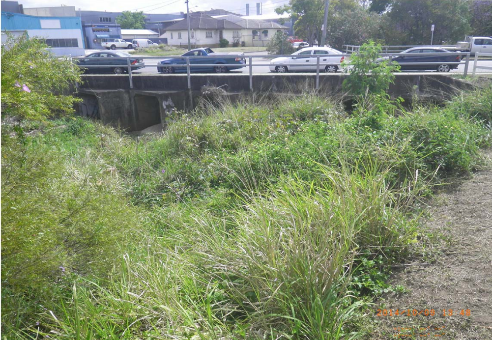
Upstream of Gladstone Road Culverts
