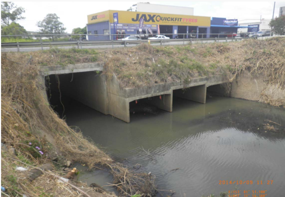
Downstream of Wynnum Road bridge/culverts
