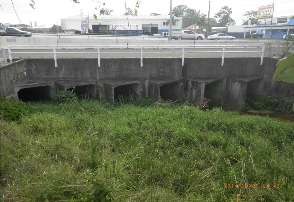
Upstream of Beaudesert Road Culverts
