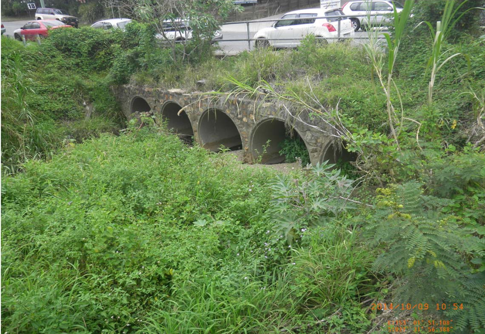
Upstream of Lucy Street Culverts
