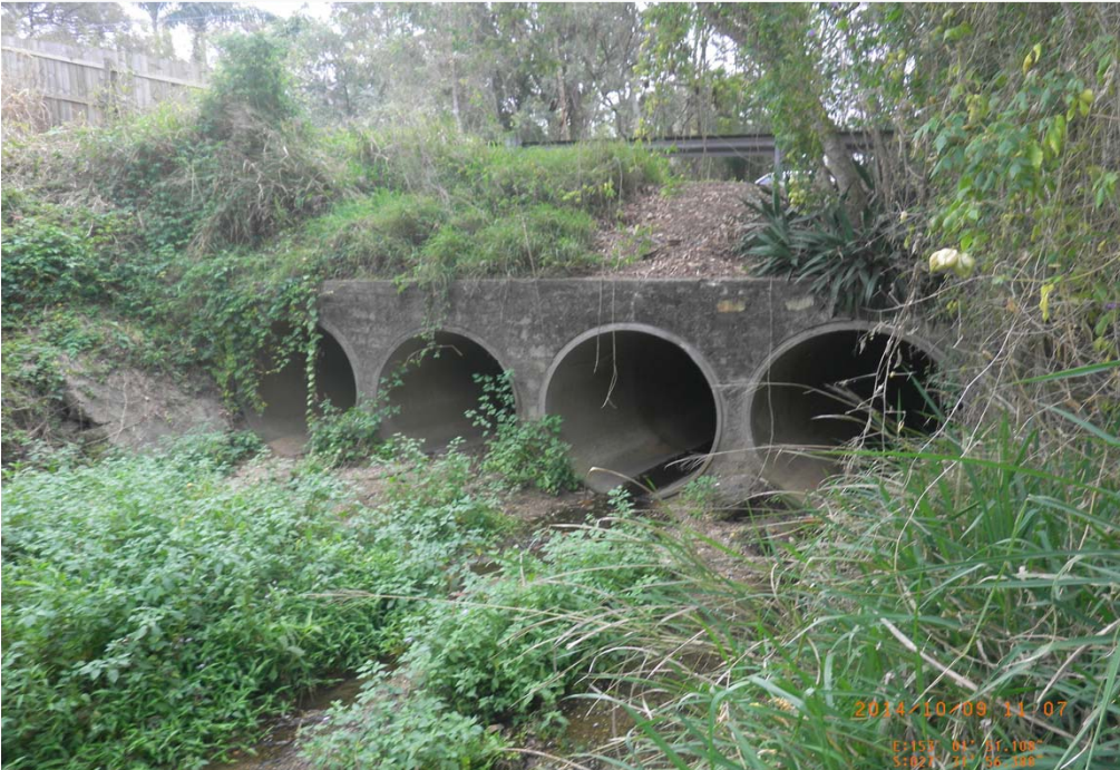
Downstream of Gow Street Culverts
