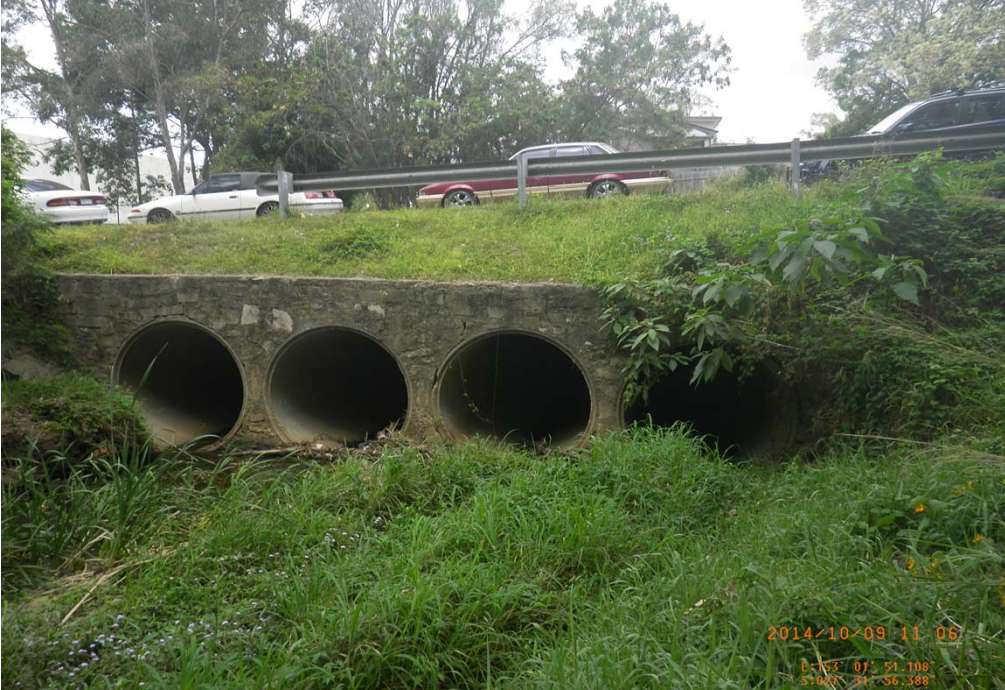
Upstream of Gow Street Culverts
