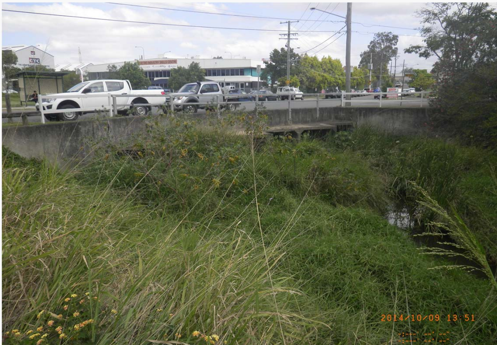
Downstream of Gladstone Road Culverts
