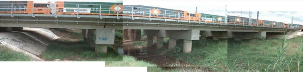
Downstream of Railway Bridges (from previous Report)
