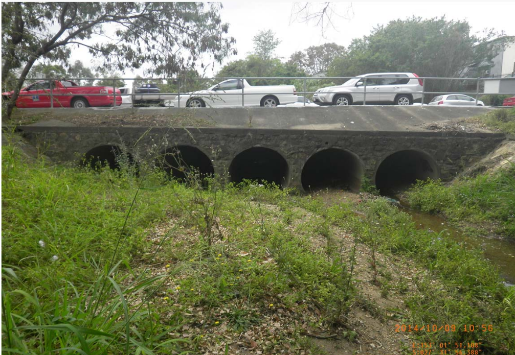
Downstream of Lucy Street Culverts
