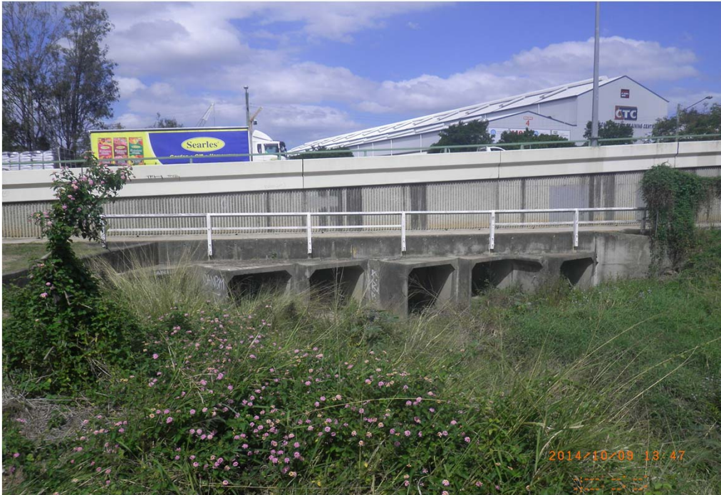
Downstream of Beaudesert Road Culverts
