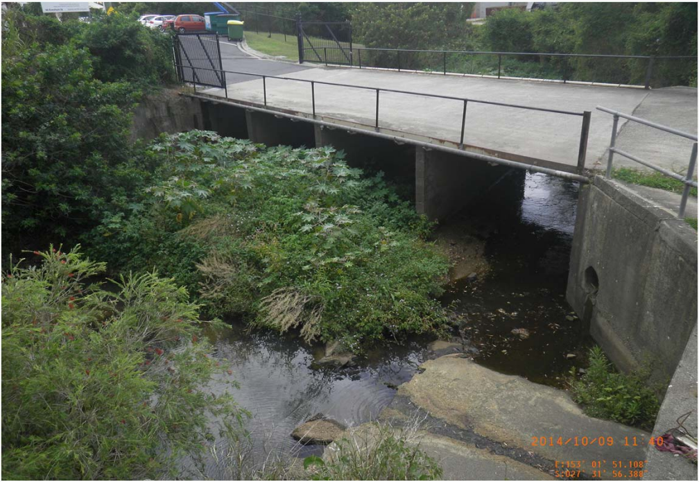
Exit of Evesham Street Crossing
